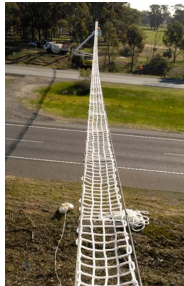
Rope bridge installation, Hume Highway
