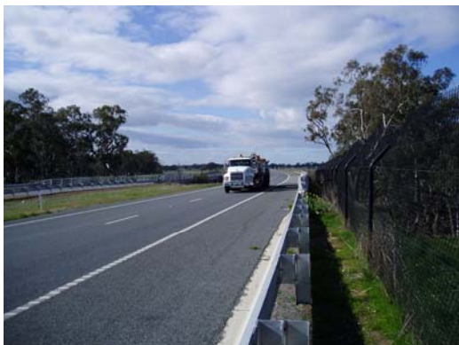
Truck on Goulburn Valley Freeway, near Murchison Photo: Rodney van der Ree
