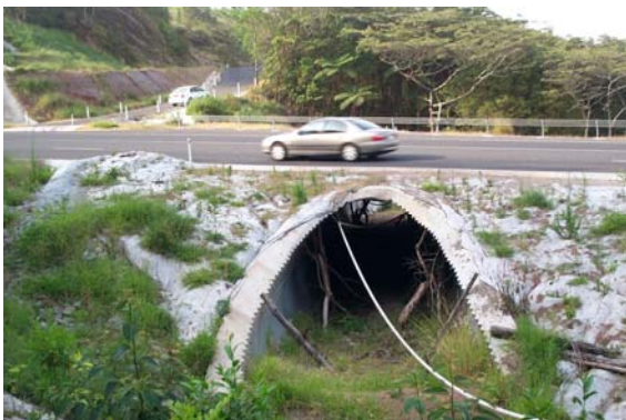
East Evelyn Road culvert, Atherton Tablelands, N. Queensland Photo: Rodney van der Ree
